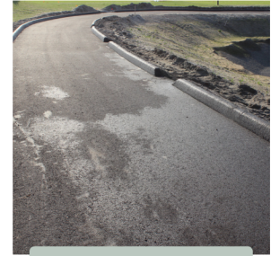
CART PATH PAVING
