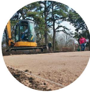
Tee Box Construction
