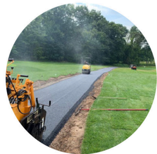
Cart Path Paving
